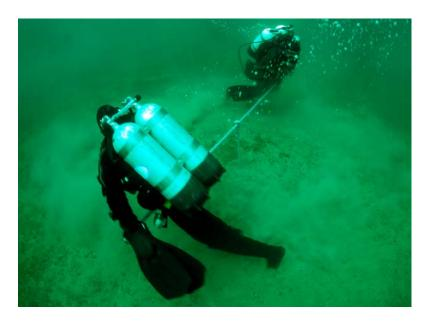
Figure 14. Screwing mooring anchors into the lakebed. Photo by Tamara Thomsen.
